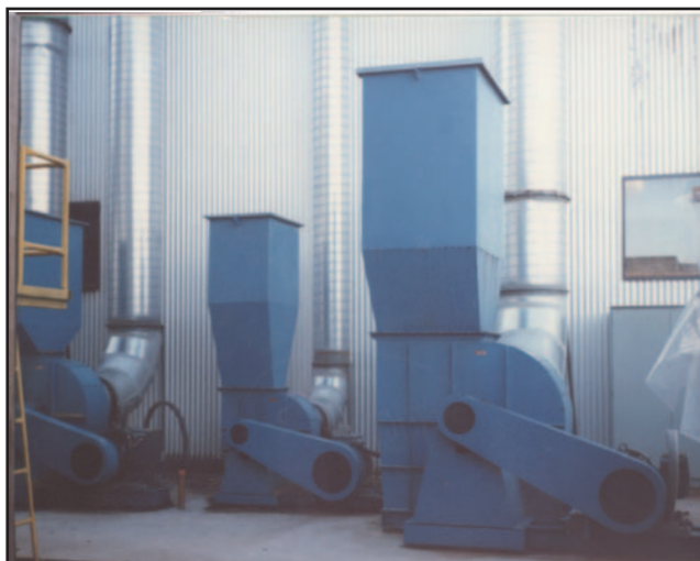
MVZ 340 (75kw), MVX 340 (55kw) and MVX 240 (30kw) Fans, Arr. 1 c/w discharge silencers
